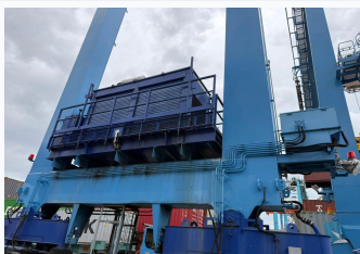
STS Gantry Crane Rehabilitation
