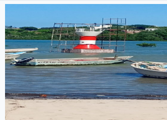
Offshore Beacon Erection
